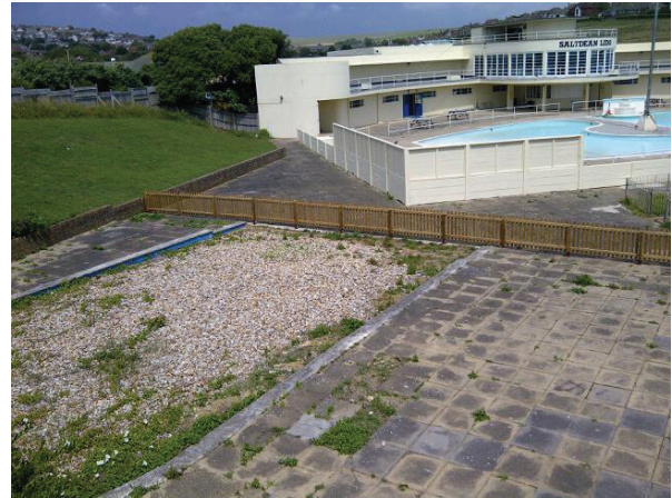
Paddling pool filled with gravel and fenced off.
