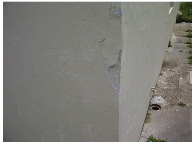
Rear sections to the lido building containing the library and community centre. Note cracks, rotten window frames and disrepair across the entire building, now simply painted over!
